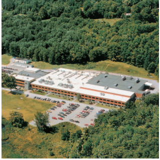
Peterborough Plant (USA)
