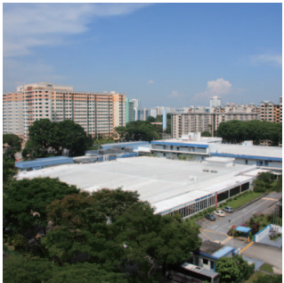
Chai Chi Plant (Singapore)
