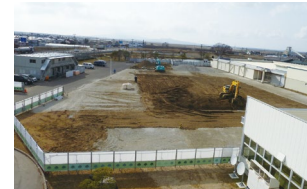
Ground concrete reused as gravel (white areas) (September–October 2018)
