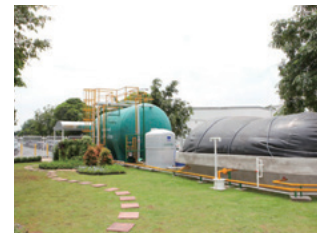
Biogas generation equipment
