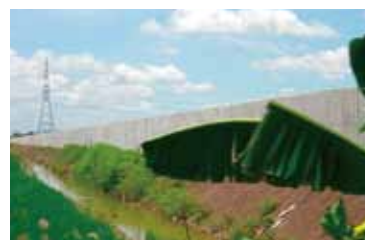
Embankments constructed around Bang Pa-in Plant, Thailand
