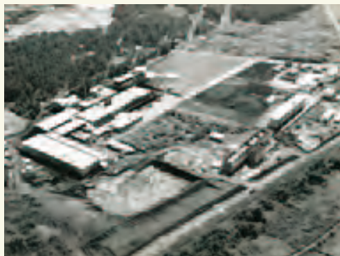
Expansion work on the Karuizawa Plant in the 1960s
