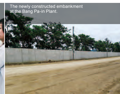
Employees unable to return to damaged homes take temporary shelter at the new bearing plant; Employees living in temporary shelters continue daily work and assist with anti-flooding countermeasures.
