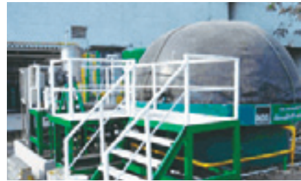
Biogas generation plant at Lop Buri Plant, Thailand
