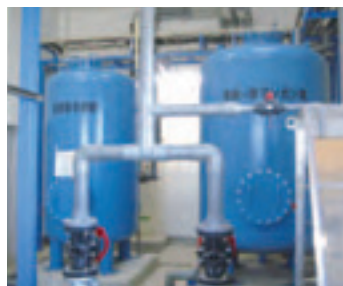
Filtration system for effective use of spring water
