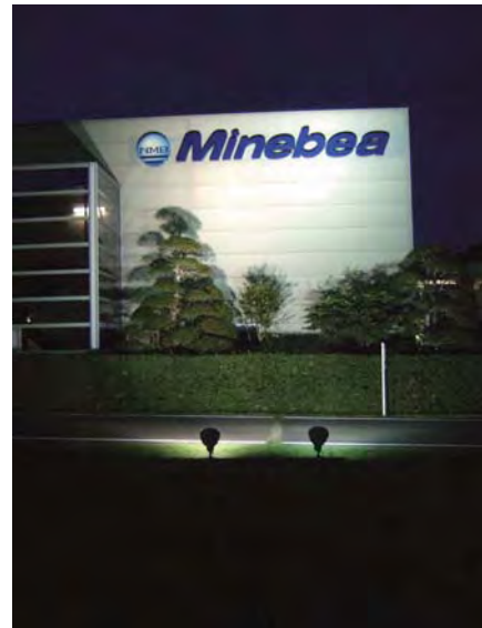
Hamamatsu Plant with lights turned on The lights and some other light in the plant were turned off from 8 pm to 10 pm on June 21st and July 7th
