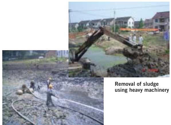
Cleaning of the river bed following sludge removal
