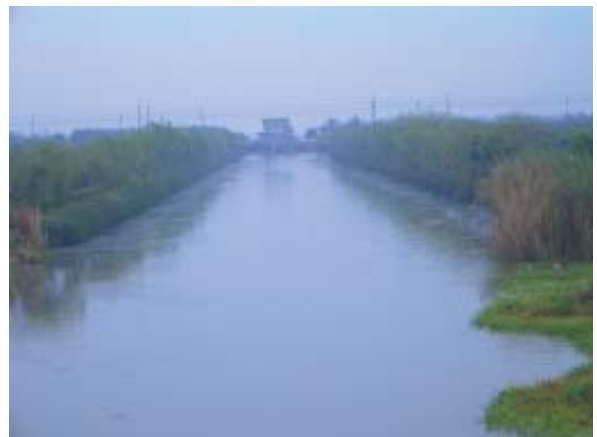
A local river after completion of dredging and planting of greenery
