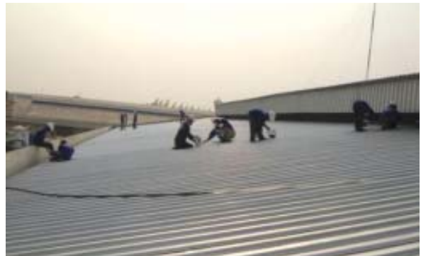
Workers coat the roof of the Rojana Plant with heat-resistant paint
