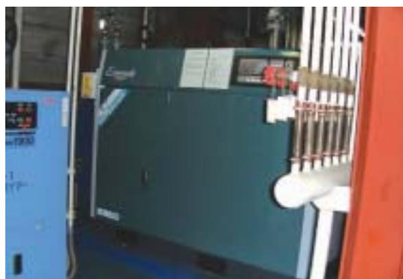
New compressors with inverters (Hamamatsu Manufacturing Unit)
