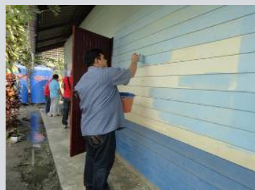
Painting the exterior walls of a rebuilding nearby school (Thailand)
