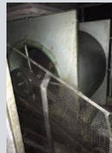
Old large belt-drive fan
