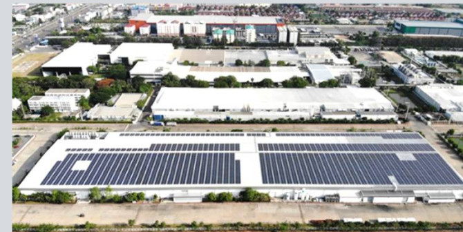
Bang Pa-in Plant
