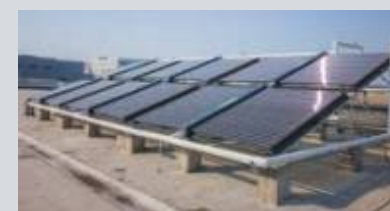
Solar hot water equipment (Wuxi·China)
