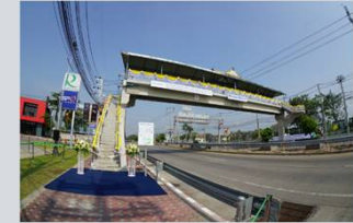
Overpass on the road in front of the Loburi Plant ( Thailand)
