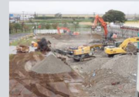
Crashed Concrete was reused around the new building and on the base of paved roads (Akita Business Division)
