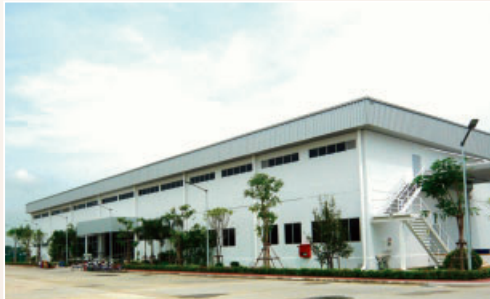
Outside view of the new cutting and pressing process factory
