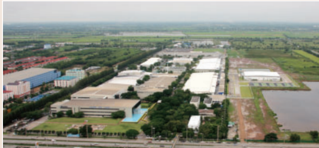
Entire view of the Bang Pa-in Plant
