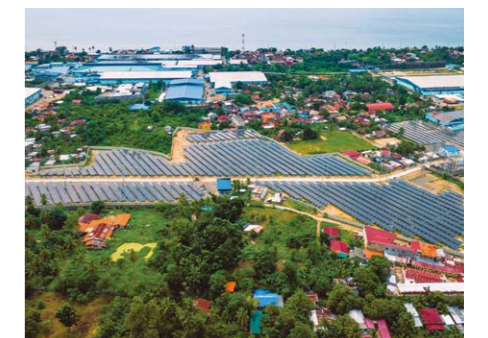
Solar power generation systems at the MITSUMI Cebu plant
