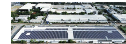
Solar power generation at Bang Pa-in Plant
