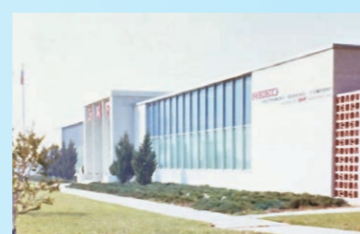
The U.S. Reed Instrument Corp. (Currently NHBB Chatsworth Plant)
