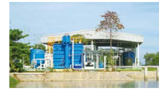
Rainwater basin and rainwater recycling equipment at the Bang Pa-in Plant in Thailand
