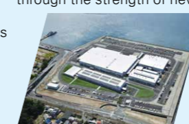
Hiroshima Plant of U-Shin Ltd.
