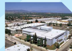
Reed Instrument Corp. of SKF, Inc. (the present Chatsworth Plant of New Hampshire Ball Bearings, Inc.)
