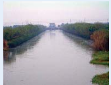
A local river after a dredging project supported by the Shanghai-Minebea Lake Dianshan-hu Environmental Protection Fund
