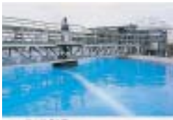
Wastewater treatment facilities at a Minebea plant in Thailand
