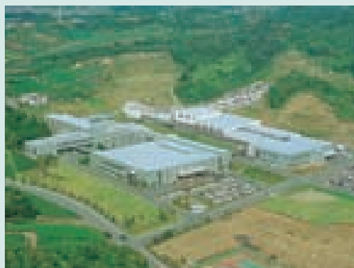
Hamamatsu Manufacturing Unit, the parent plant for switching power supplies and other electronic devices and components
