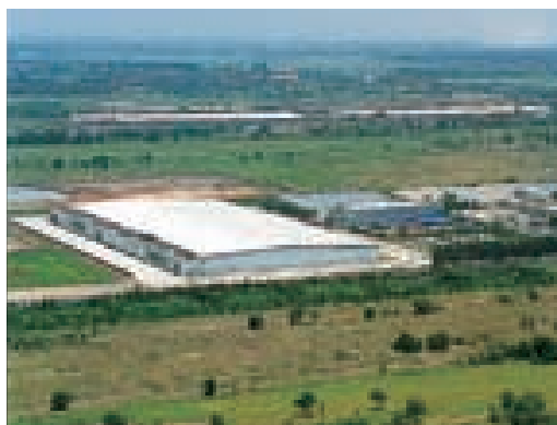
New facility for fluid dynamic bearings and HDD spindle motors, Bang Pa-in, Thailand
