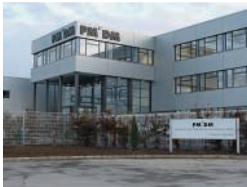
New facility built for Precision-Motors-Deutsche-Minebea-GmbH
