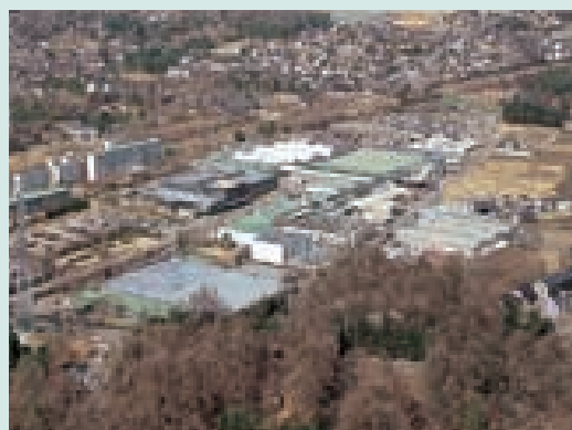
Karuizawa Manufacturing Unit, the parent plant for bearings, small motors and other machinery components
