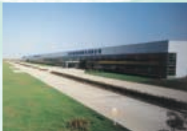
The Shanghai Plant of Minebea Electronics & Hi-Tech Components (Shanghai) Ltd.
