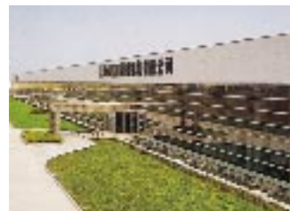
Minebea's newest plant, in Shanghai
