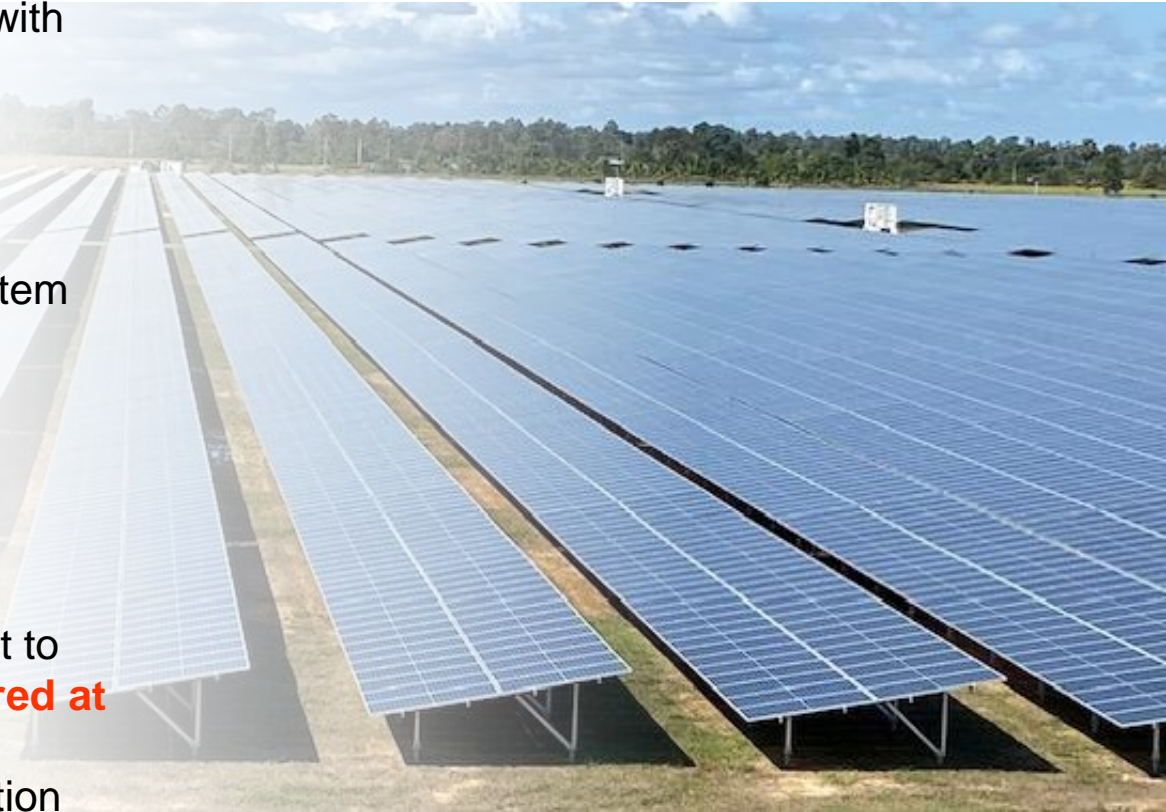
Solar power system already installed by SchneiTec
