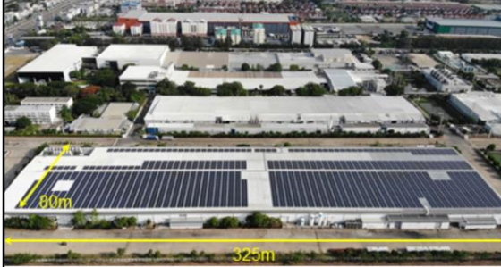
Bang Pa-in Plant
