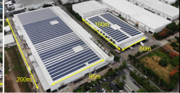
Lop Buri Plant
