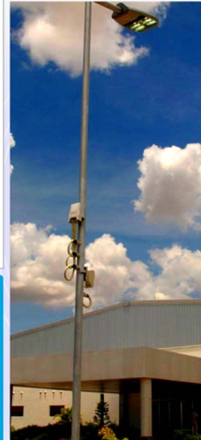
Smart LED street light
