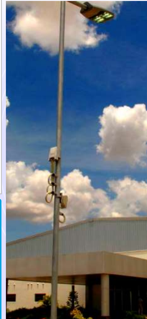
Smart LED street light
