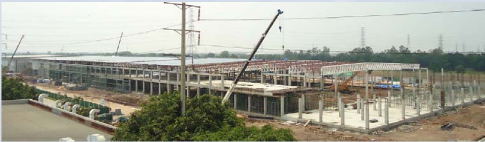
New ball bearing plant currently under construction (Bang Pa-in, Thailand)
