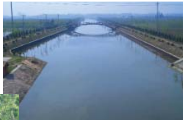
Riparian works funded by the Shanghai–Minebea Environmental Protection Fund
