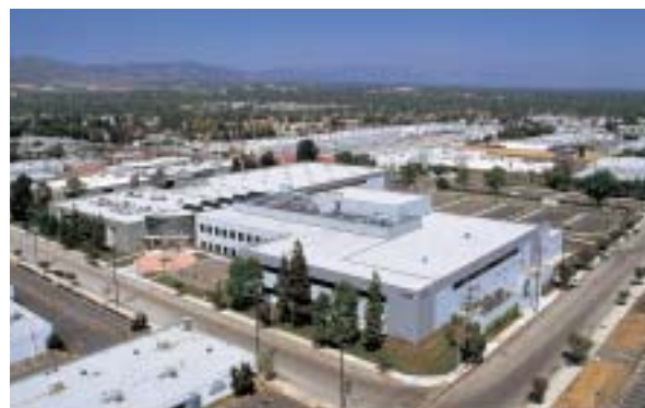
NHBB’s Chatsworth Plant
