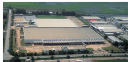
New Ban Wa Plant (Thailand)
