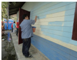
Painting the school walls
