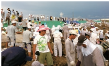
The levee installations and employees that protected the Bang Pa-in Plant from flooding.
