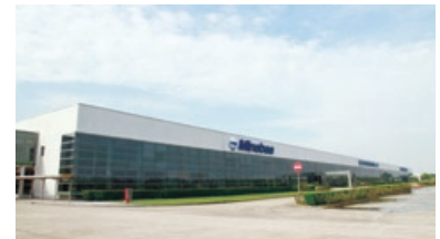
1994 Establishment of Shanghai Plant
