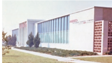
1971 Commencement of production in USA
