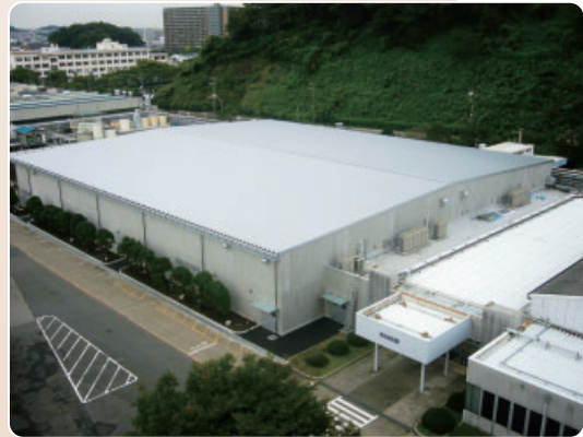
A view of new factory building in Fujisawa Plant
