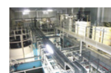
Fujisawa Plant's wastewater treatment facility
