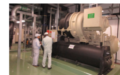
Centrifugal chiller installed in the Xicen Plant, China
