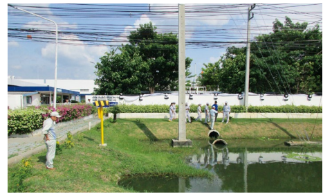
Inspection of drainage at the Ayutthaya Plant, Thailand
